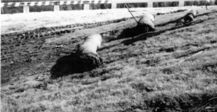
FIGURE 12. Grass carpets introduction into the landfill slopes
