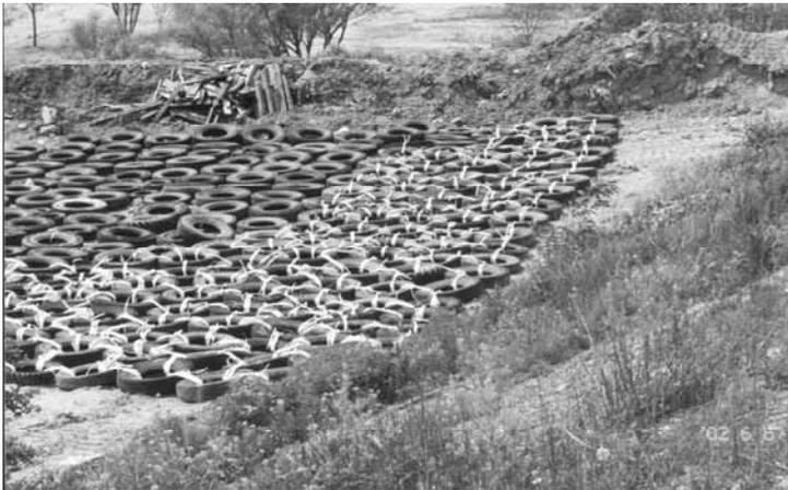
FIGURE 2. Preparation of mattresses made of used tires to reinforce of western landfill slope
