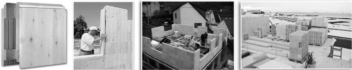
Picture. 1 Timber module used for house self-assembly and house construction using the system designed by Steko company.
