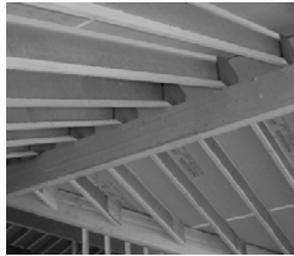
Picture. 4 Joining the rafters resting on purlin in Masonite system
