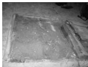
Drawing 5. Floorings' layout: a,b- flooring from Ostrowy Tuszowskie with the sand layer visible, c- forged nail that joined Kolbuszowa panel with the blind floor
