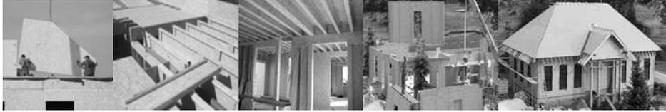
Picture. 1 House construction using Kronopol system.
